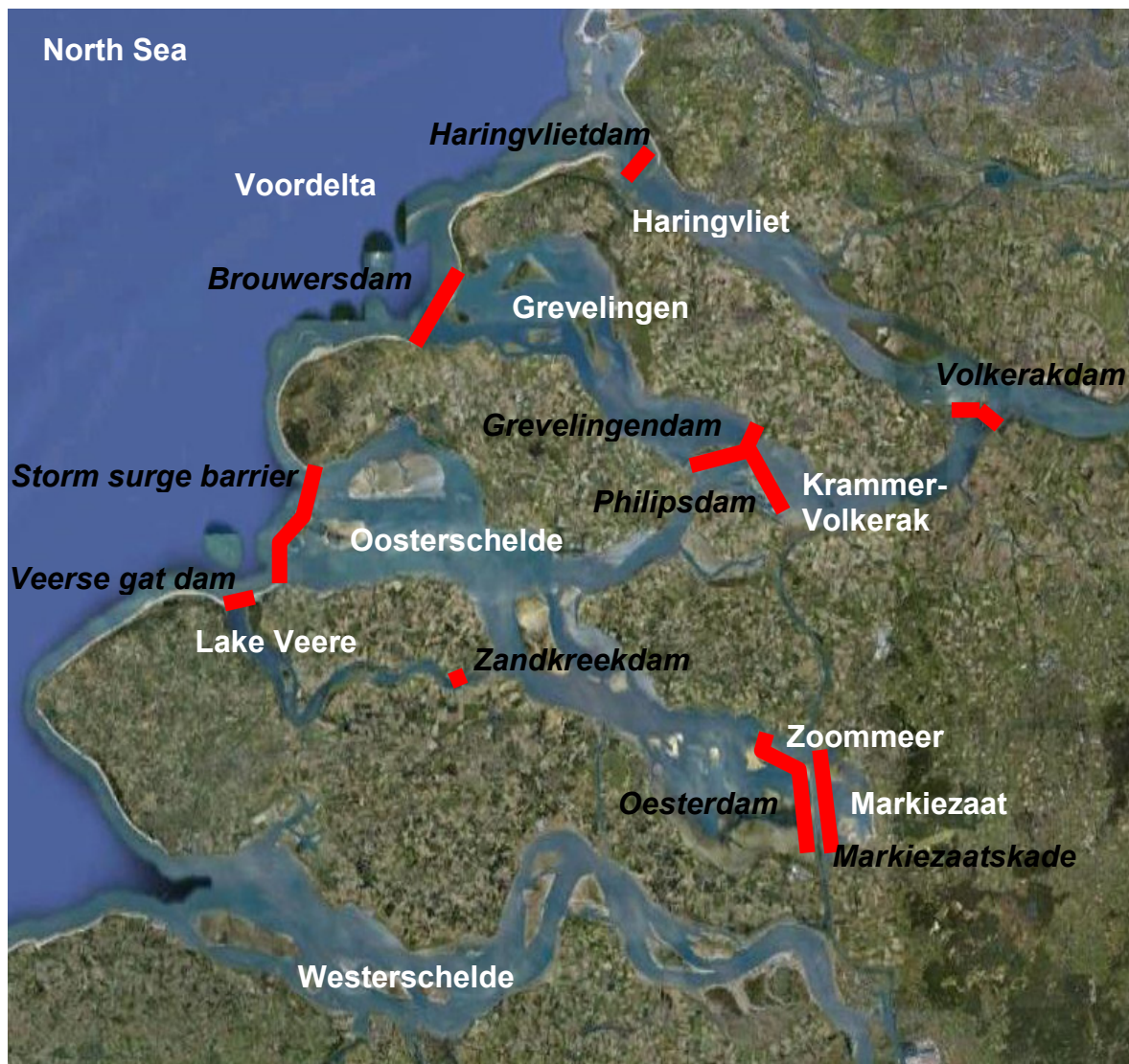
Figure 1. An overview of the South-Western Delta, showing the different water basins (white text) and coastal engineering works (red with black text) that are part of the Delta project.
